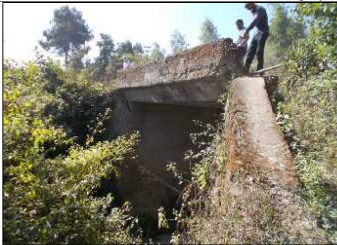
Bridge Inventory (Ch. 13.557 km)
