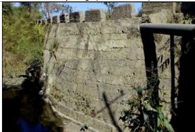
Retaining Wall at Ch. 33.325 km
