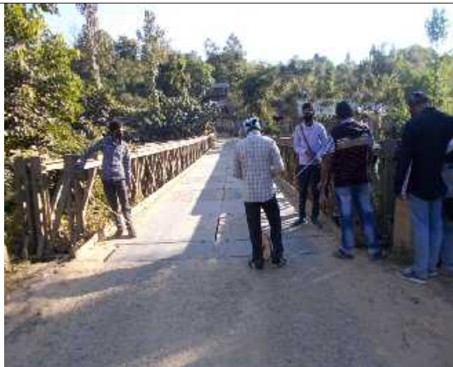
Bailey Bridge (Ch. 48.304 Km)
