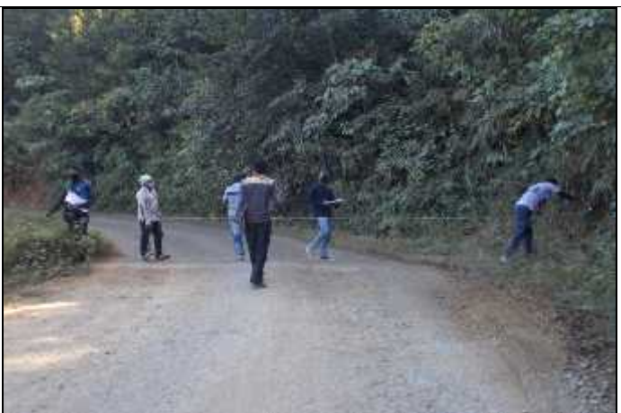
Culvert Inventory (Ch. 55.449 km)
