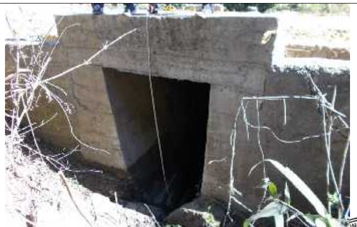
Slab Culvert (Ch. 44.482 Km)
