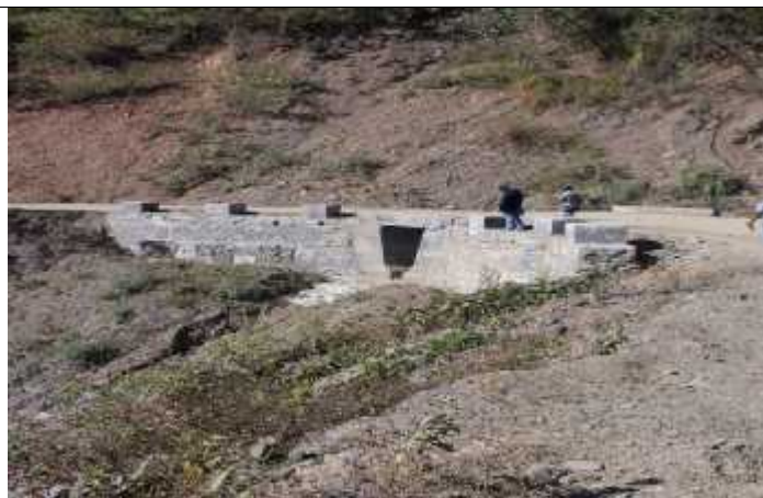
Slab Culvert (Ch. 35.494 Km)
