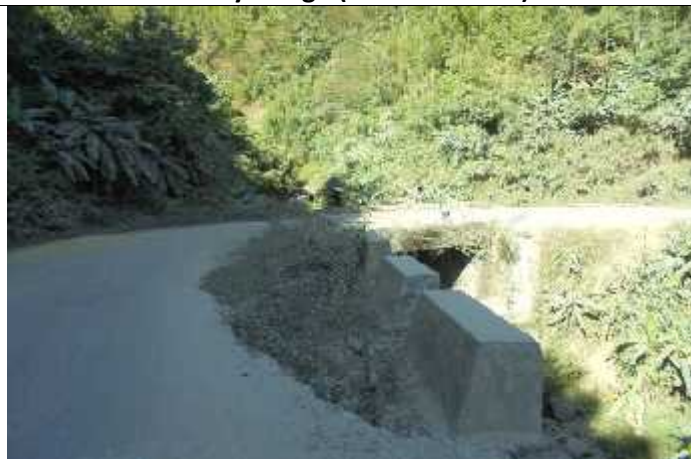
Guard Wall at Ch. 41.620 km
