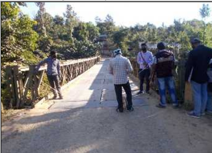
Bridge Inventory (Ch. 48.304 km)
