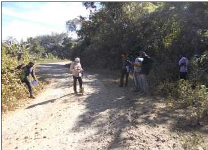
Culvert Inventory (Ch. 55.168 km)
