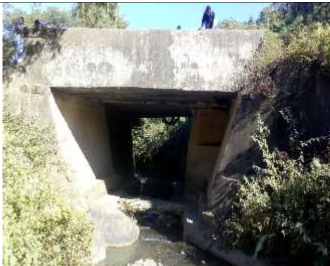
Bailey Bridge (Ch. 46.242 Km)
